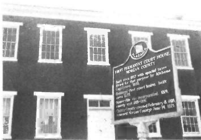
Court House, Somerville, Alabama (Not in use 1977)
